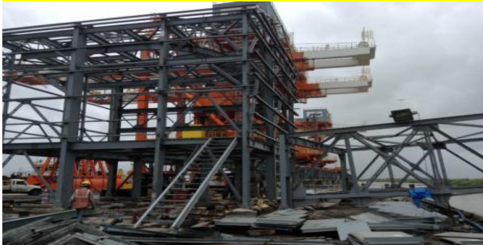
IRON ORE HANDLING STRUCTURES -JSW
