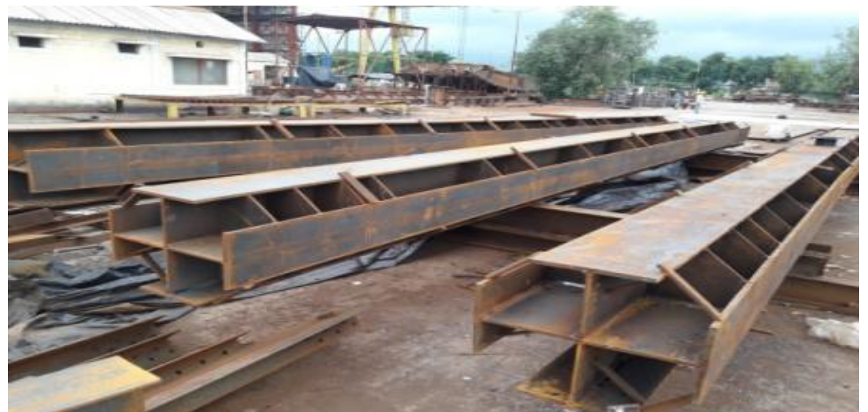
COAL HANDLING STRUCTURE - DOOSAN PROJECT
