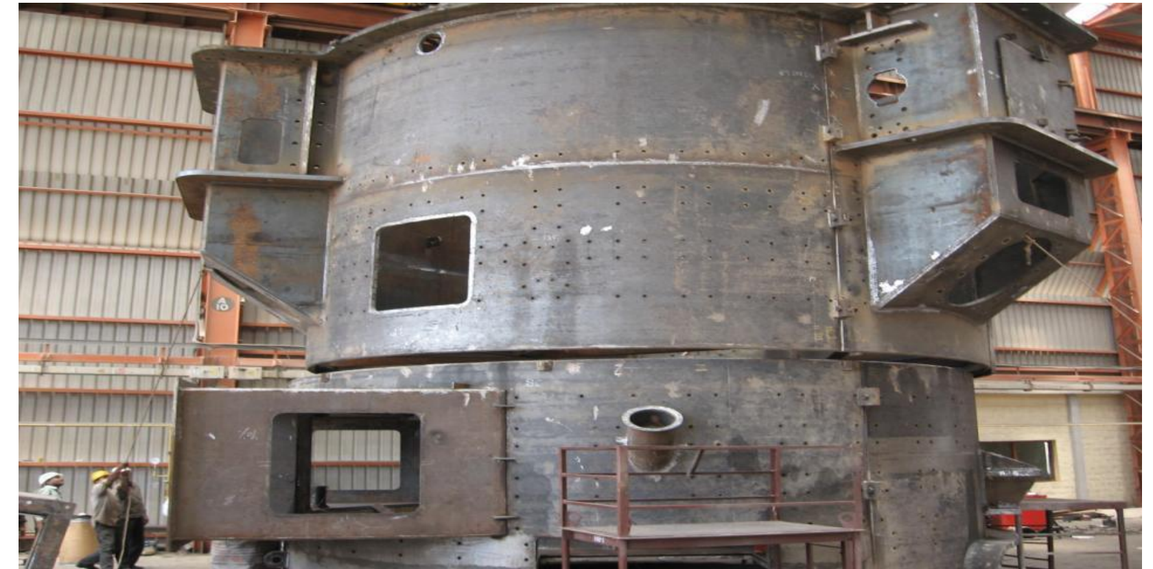
Top & Middle part of Raw Mill Housing
