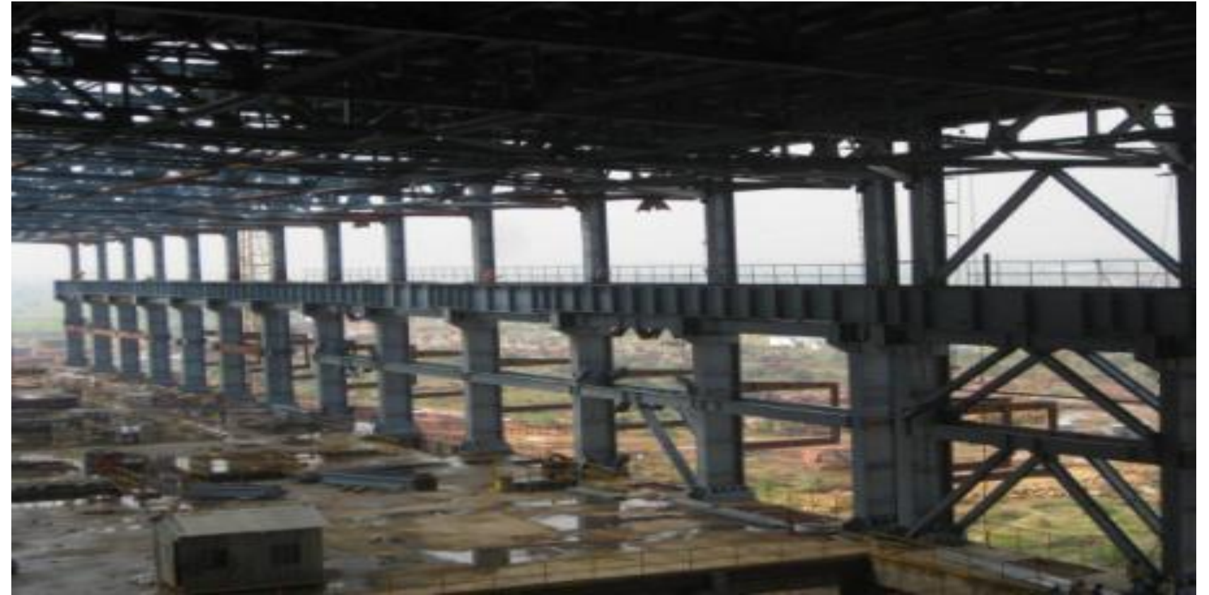
JAYPEE NIGRIE SUPER THERMAL POWER PLANT STRUCTURE
